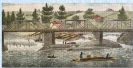
Drawing from 1835 showing the wooden truss bridge on stone piers. Courtesy Pejepscot History Center.
