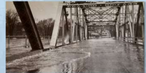
The record setting 1936 floodwaters reached the deck of the Frank J. Wood Bridge. Courtesy Maine DOT.
