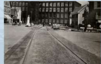
In 1932 the trolley line was reconstructed in the north end of downtown Brunswick as part of the approach to the new Frank J. Wood Bridge. Courtesy of MaineDOT.
