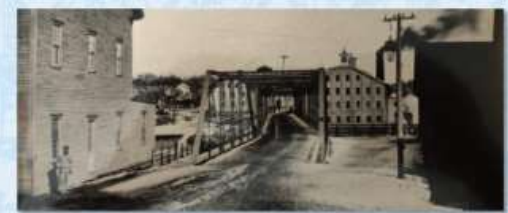
1889 iron bridge and its angled roadway. Courtesy Pejepscot History Center.
