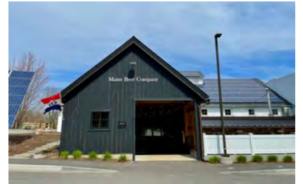
Figure 2.120-A. Examples of the Workshop-Warehouse Building
