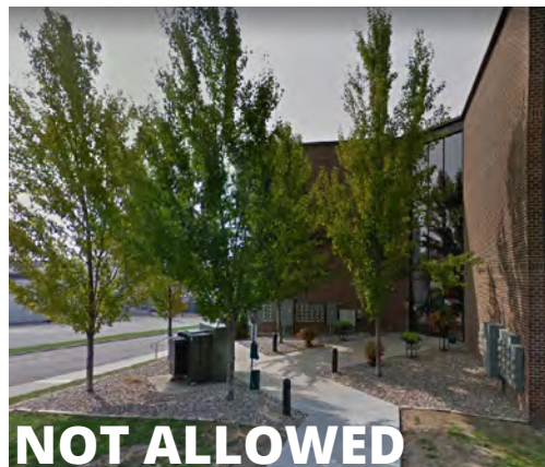
Figure 8.40-I. Examples of Poorly Located Utility Appurtenances on Primary Streets
